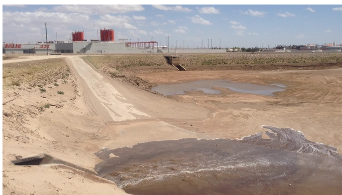
Basins at the Jonathan Rogers Plant will soon take in water from the Rio Grande.
